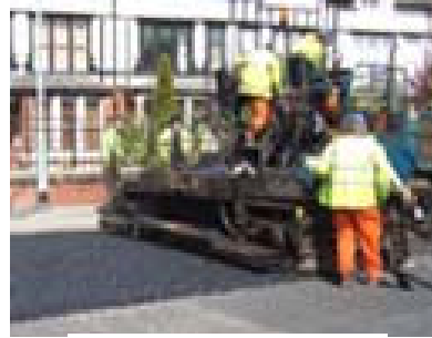
Highway repairs Leeds
